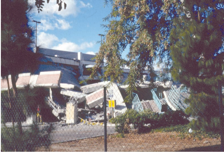
FIGURE 2.9 Parking garage collapse, Northridge, California, 1994. Photo credit, Susan Cutter.
