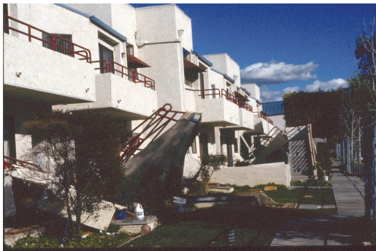
FIGURE 2.8 Apartment building collapse, Northridge, California, 1994. Photo credit, Susan Cutter.
